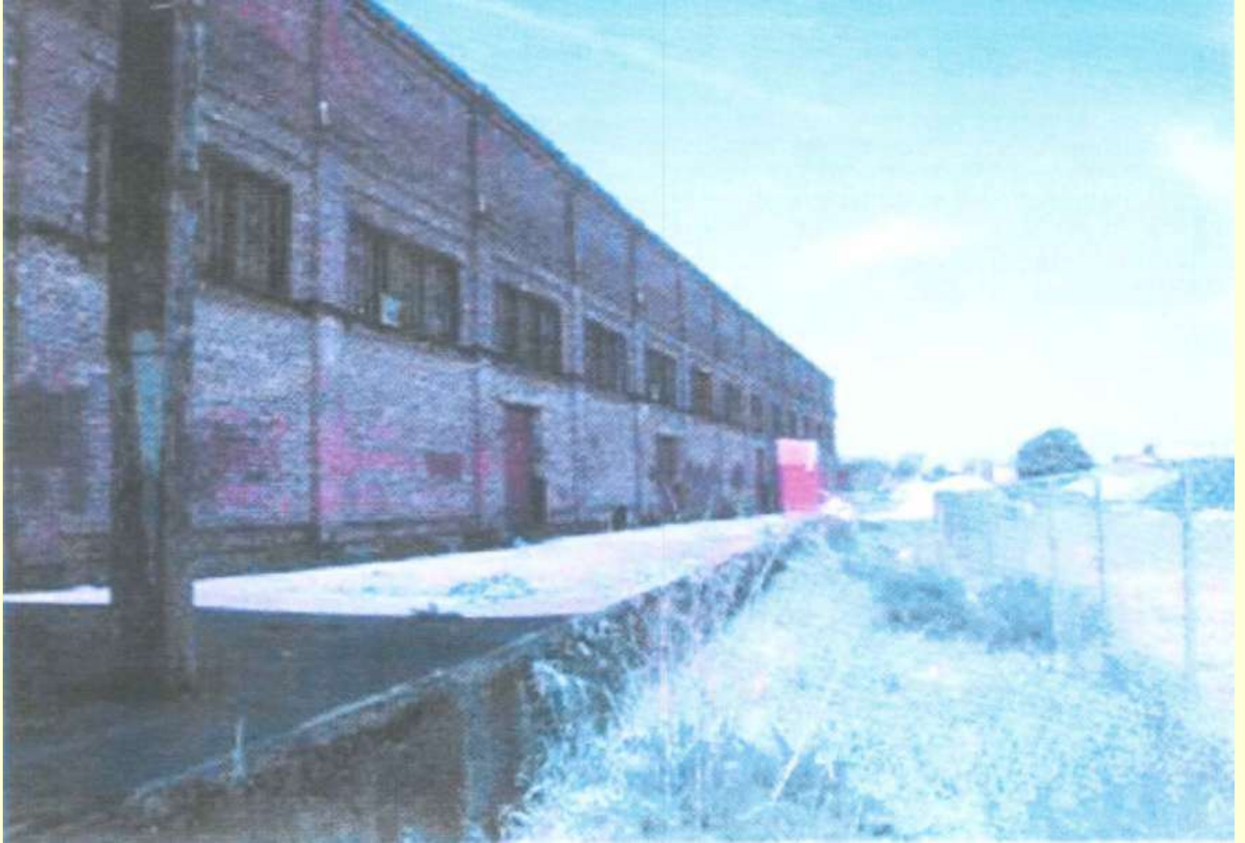
East Facing Wall & Loading Dock
