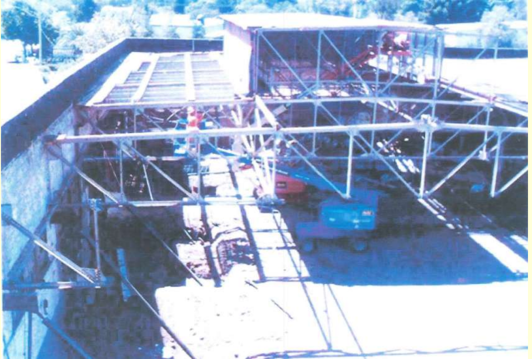
Demolition Partially Complete
