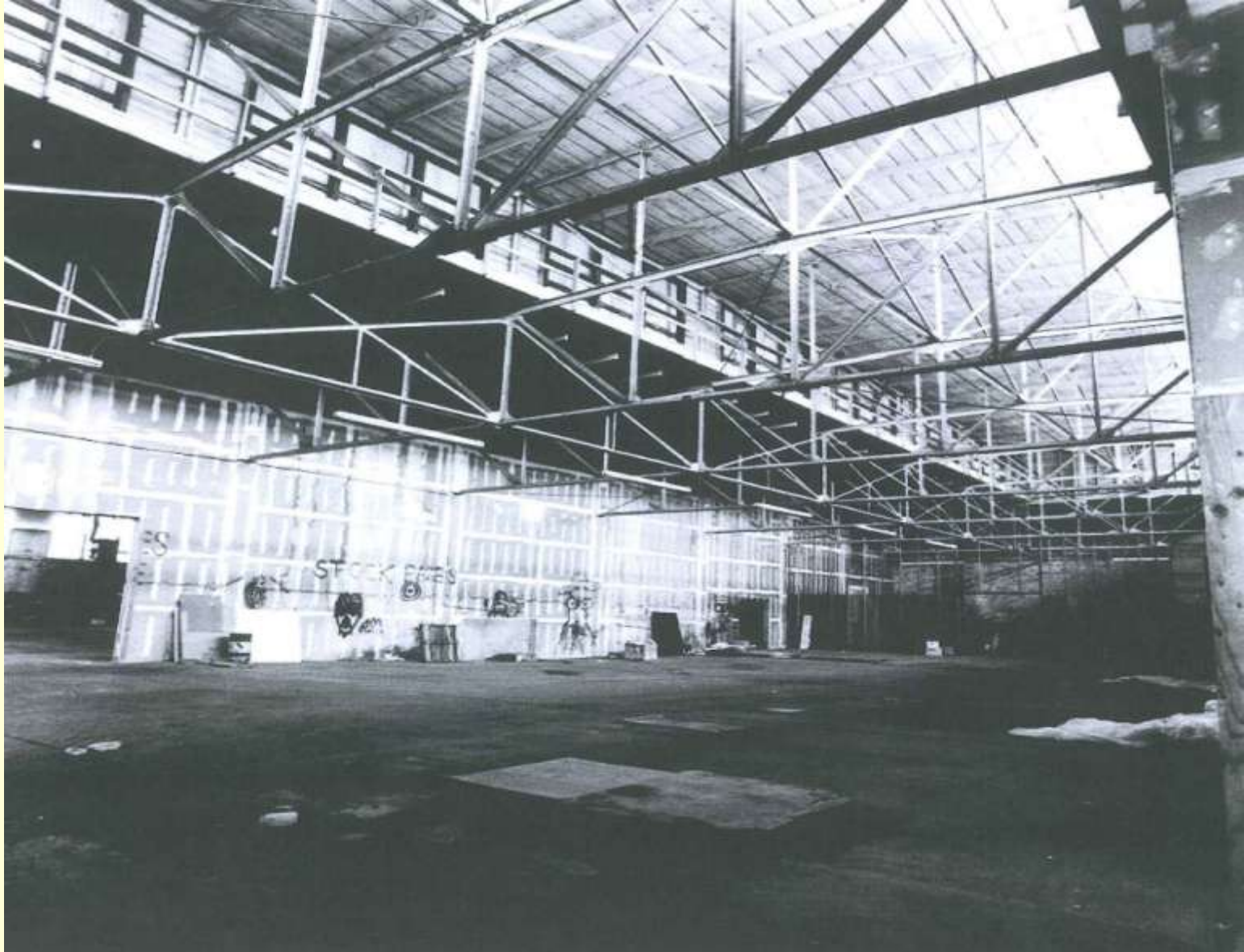
3 West Third Street Cannery Interior
