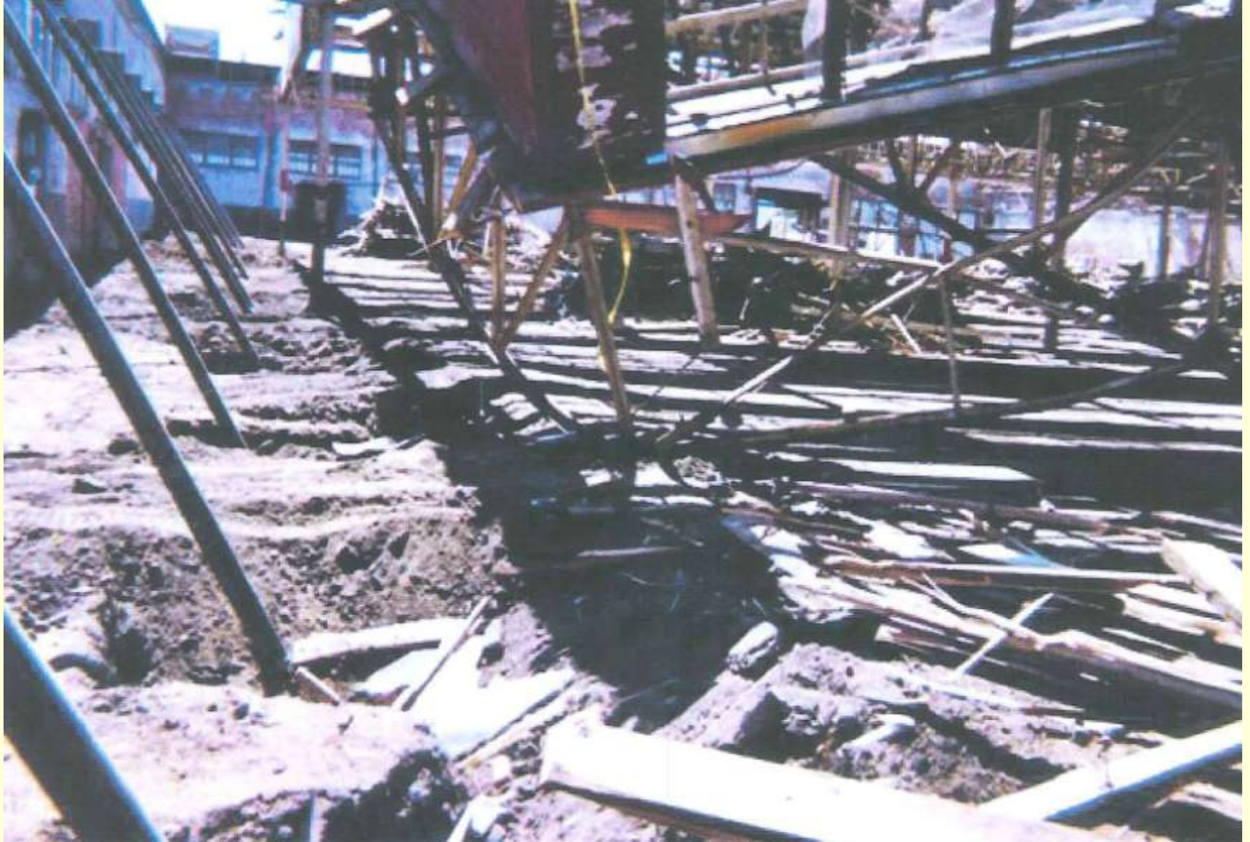
Braced Walls and Demolition
