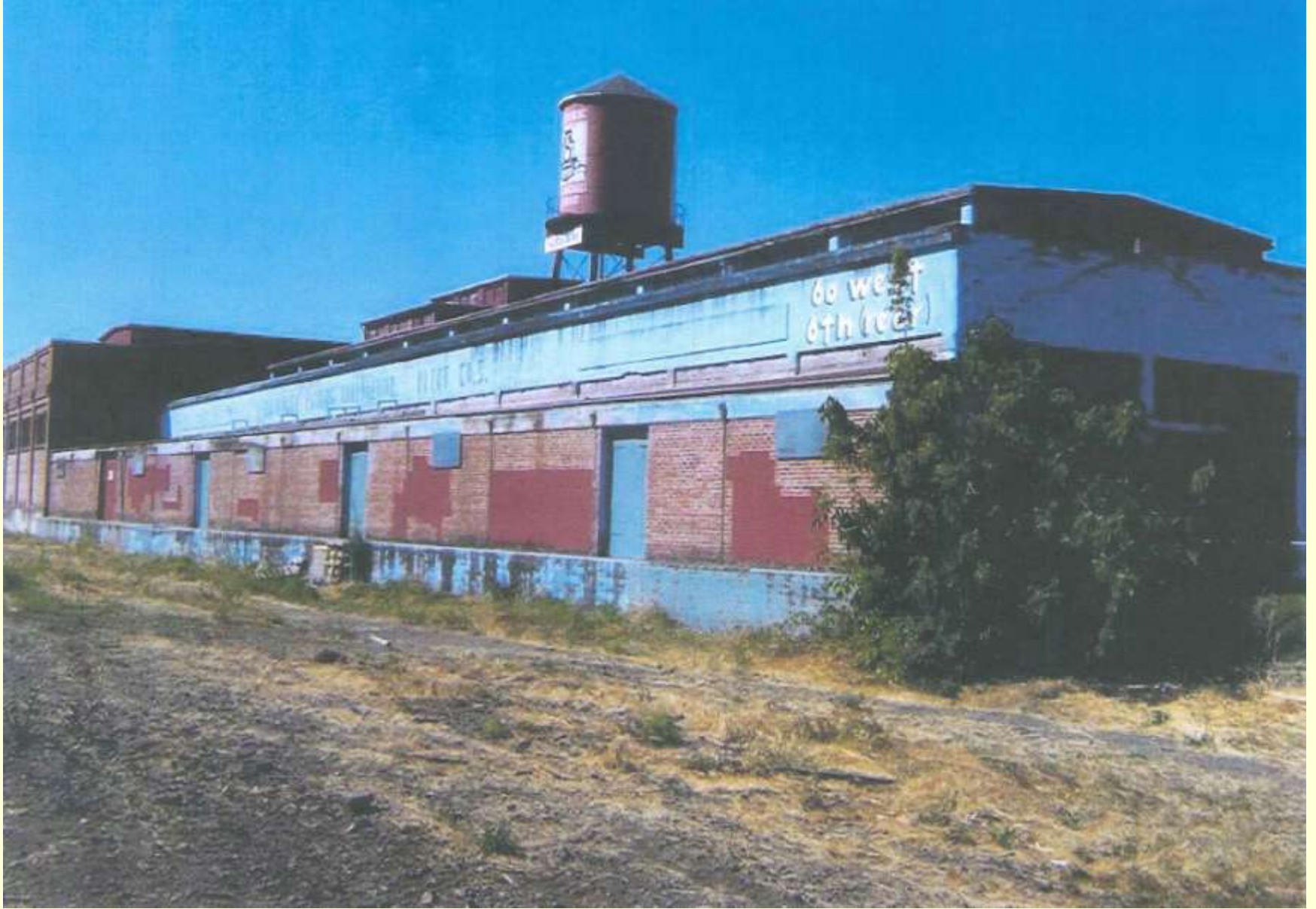
60 West Sixth Street Cannery (Plant 5)
